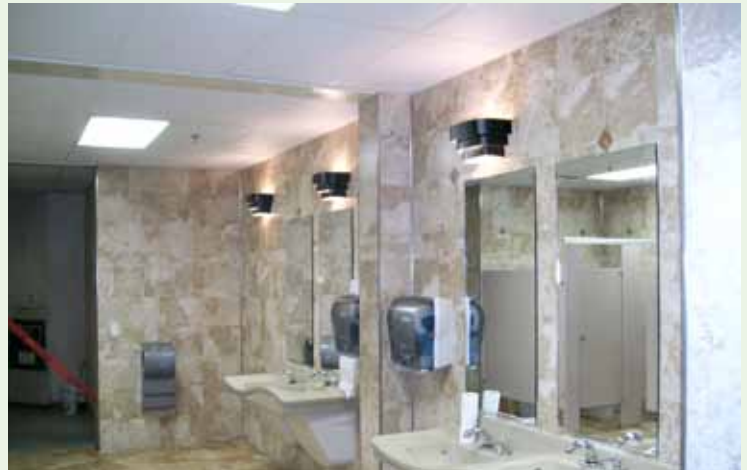
Men's locker room after
